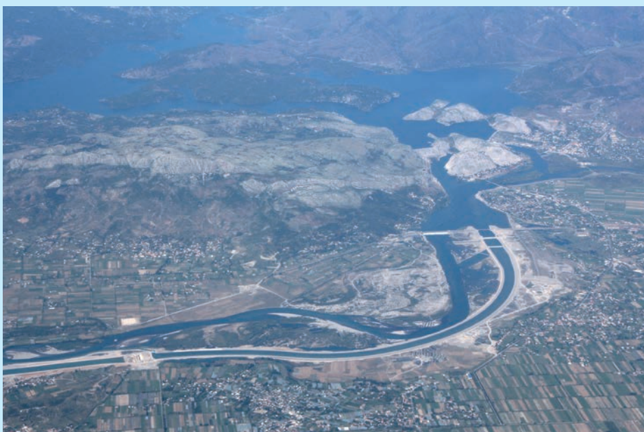
Aerial photograph of Ashta power plant
